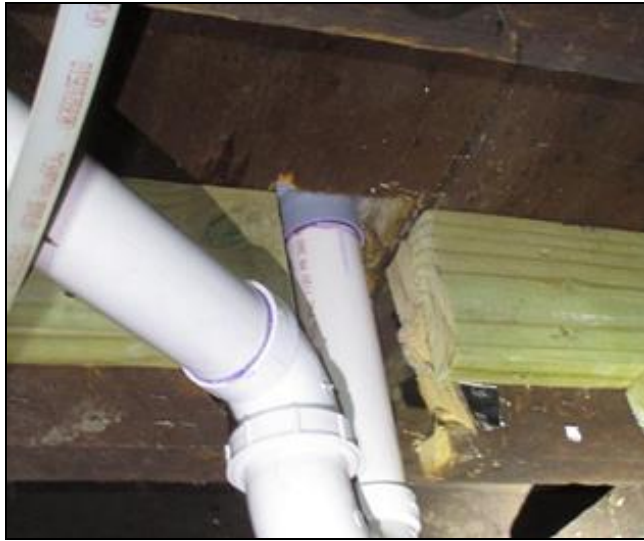
7.3 Item 1(Picture) When main floor bath was remodeled, a floor joist was cut completely. While chances of future floor failure are slim, the floor joist should have been properly 'boxed'
