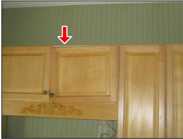
4.5 Item 1(Picture) One cabinet door is loose.
