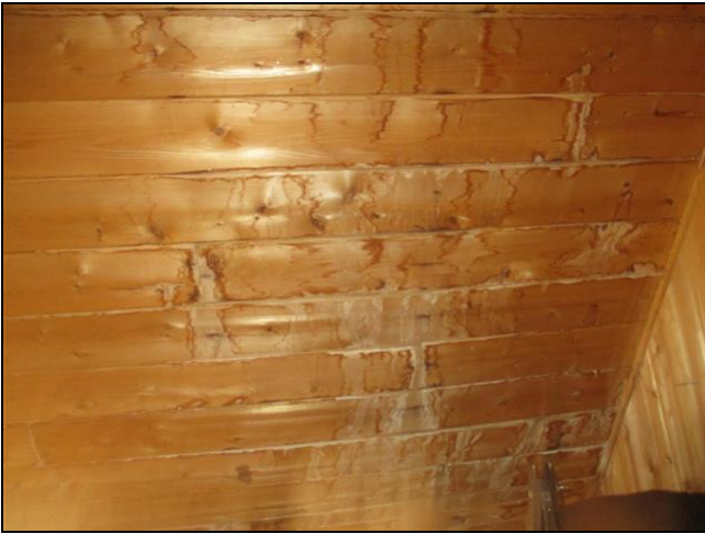
5.0.E Item 1(Picture) Ceiling is stained, likely from prior water leak.
