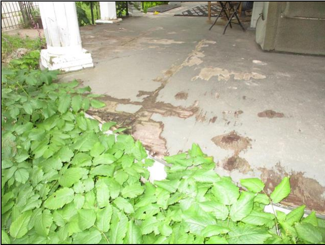
2.3 Item 3(Picture) East side porch and pillars show signs of water damage.
