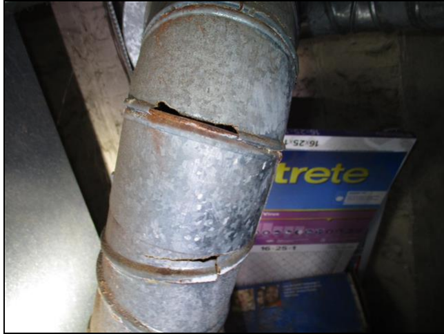
10.5 Item 1(Picture) Exhaust pipe for furnace has rotted and needs to be replaced.
