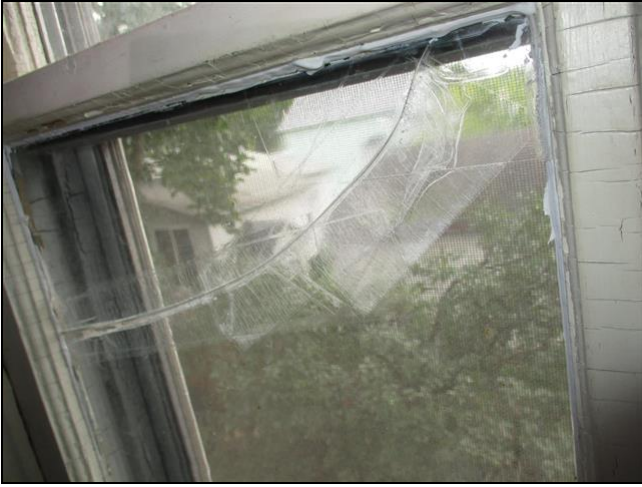
5.4.F Item 1(Picture) West facing window has broken glass.
