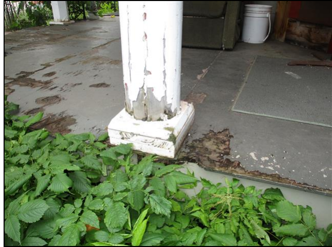
2.3 Item 2(Picture) East side porch and pillars show signs of water damage.
