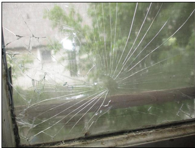
5.4.D Item 1(Picture) North facing window has broken glass.
