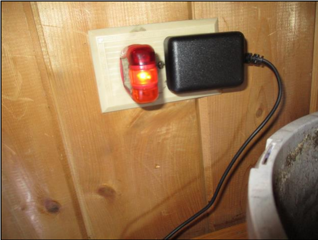
5.5.E Item 1(Picture) 3 prong outlet in this room is not grounded.
