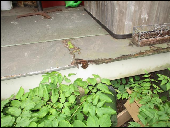
2.3 Item 1(Picture) East side porch and pillars show signs of water damage.
