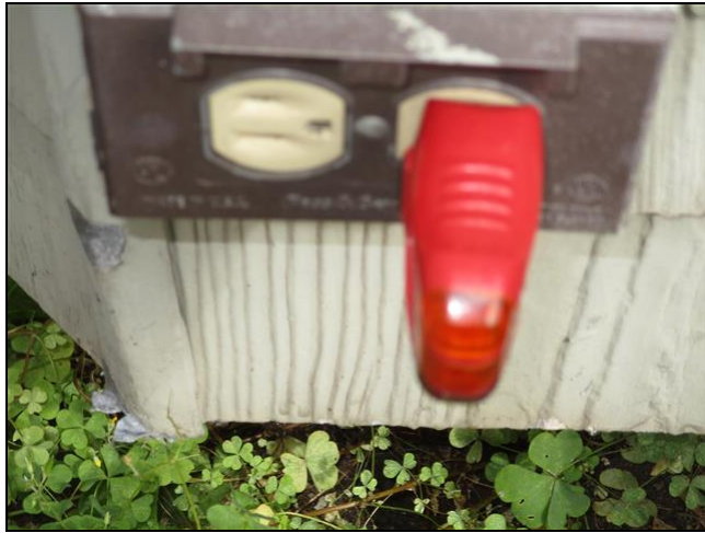
2.7 Item 1(Picture) Weatherproof cover is missing.
