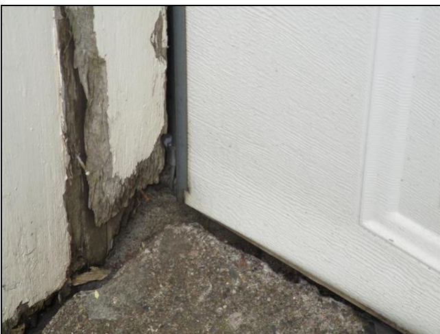
3.5.A Item 1(Picture) Evidence of water intrusion on exterior overhead door trim.
