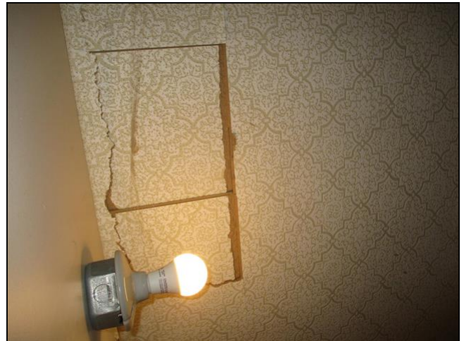
5.0.A Item 2(Picture) Ceiling tile damaged in two locations.
