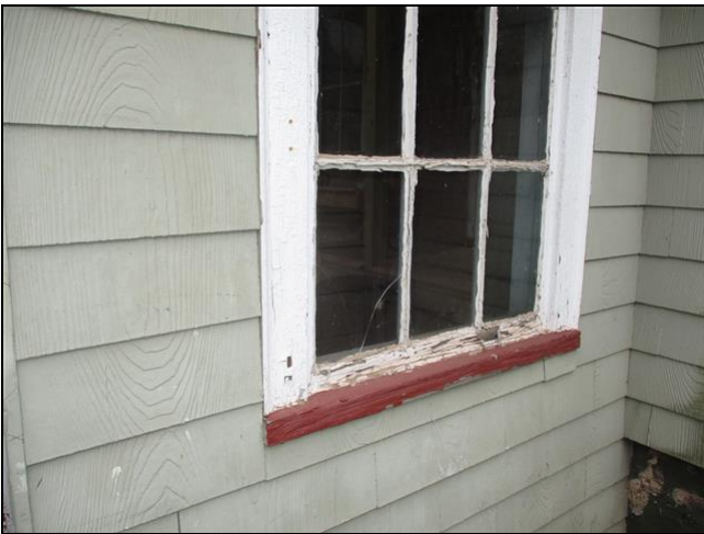
2.1 Item 1(Picture) Several windows would benefit from a fresh coat of paint to protect the wood
