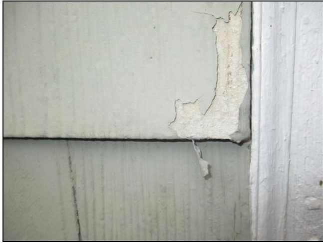
2.0 Item 2(Picture) Siding may contain asbestos, would benefit from a fresh coat of paint.
