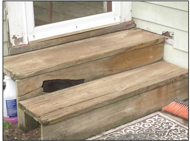
2.3 Item 4(Picture) Steps for South entry in poor condition.
