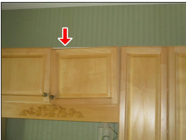
4.5 Item 1(Picture) One cabinet door is loose.
