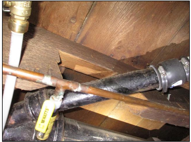
7.3 Item 2(Picture) Example of compromised floor joist that has not failed
