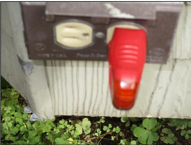
2.7 Item 1(Picture) Weatherproof cover is missing.
