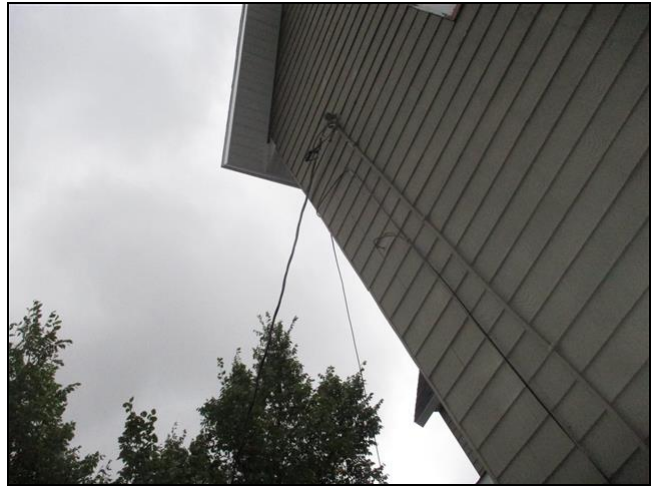
2.7 Item 2(Picture) Entrance cable is routed through trees on East side that may need to be trimmed.
