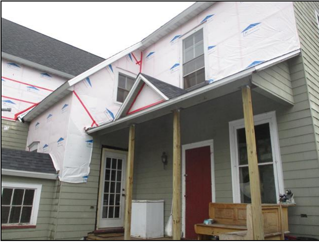
2.0 Item 1(Picture) Siding missing on North and West sides of home.
