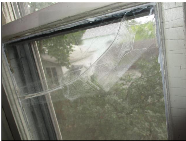
5.4.F Item 1(Picture) West facing window has broken glass.
