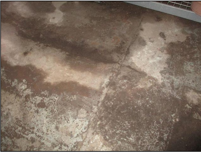
7.0 Item 1(Picture) Slab floor is main basement is damp.
