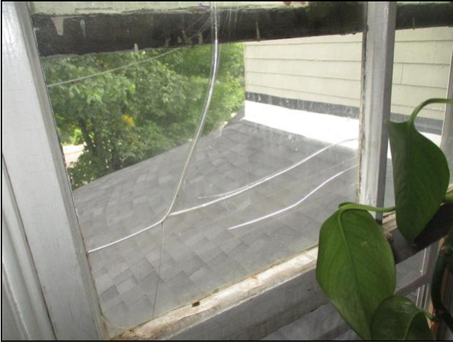
5.4.C Item 1(Picture) East facing window has broken glass.
