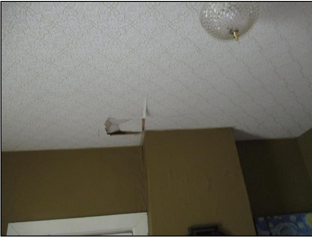
5.0.A Item 1(Picture) Ceiling tile damaged in two locations.
