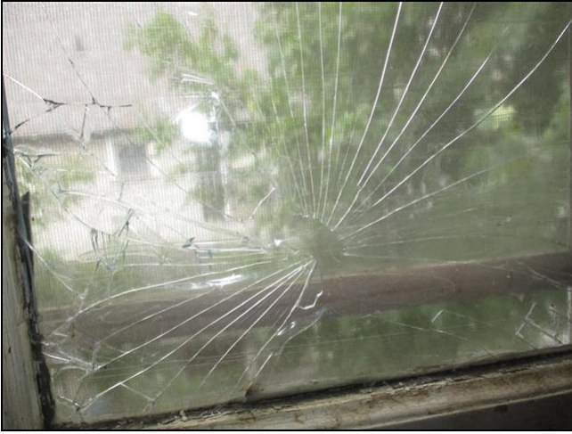
5.4.D Item 1(Picture) North facing window has broken glass.
