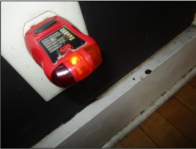
5.4.J Item 1(Picture) Receptacle on West wall is not grounded.
