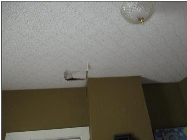
5.0.A Item 1(Picture) Ceiling tile damaged in two locations.
